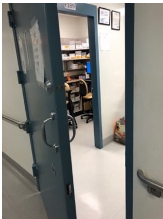
Photo 22. Pharmacy doors were not kept locked to prevent unauthorized entry (photographed on March 4, 2021).
