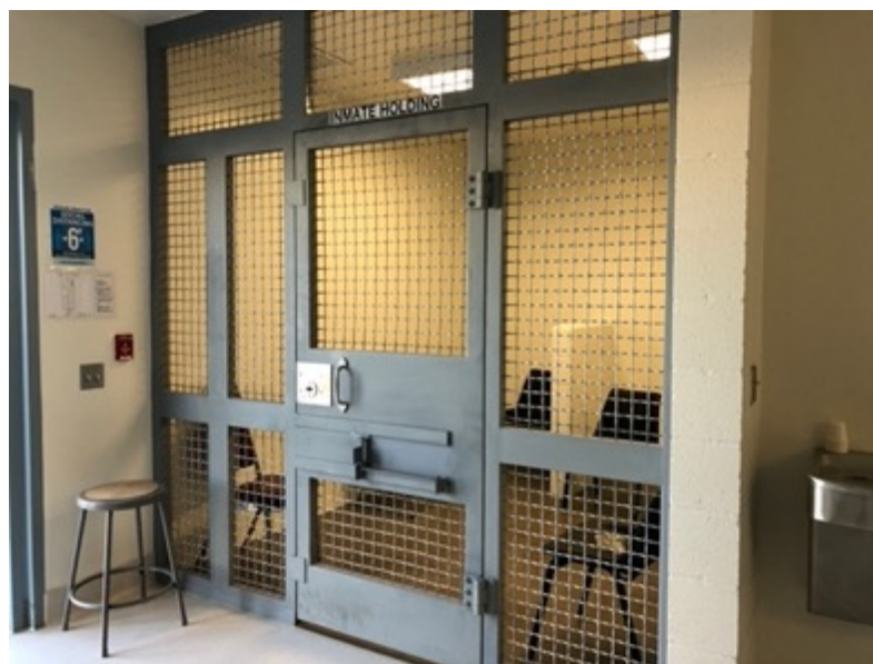
Photo 1. Indoor waiting area (photographed May 12, 2021).
