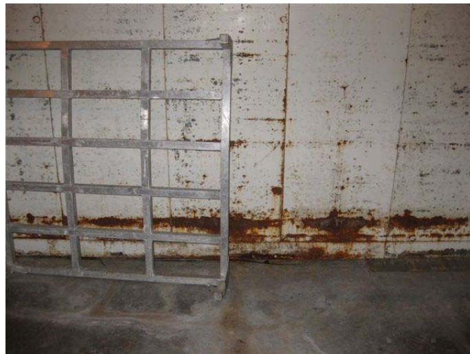
Figure 3 – Water Leakage and Rust Inside of a Refrigerator
