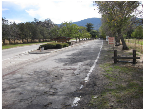
Figure 3 – CCI Road Conditions: Front Entrance. Photo: OIG October 2010
