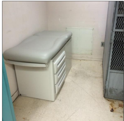
Figure 2: Inadequate exam space in the R&R clinic
