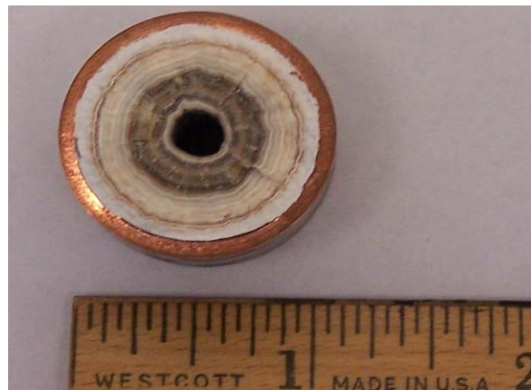
Copper pipe clogged by mineral deposits at CIM
