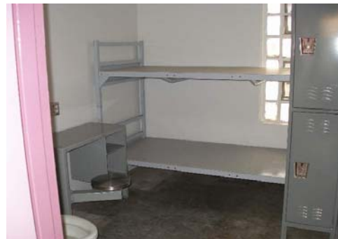
Living unit cell after renovation.
