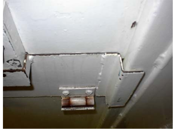
Food tray slot altered by the plant operations staff to prevent gassing assaults.
