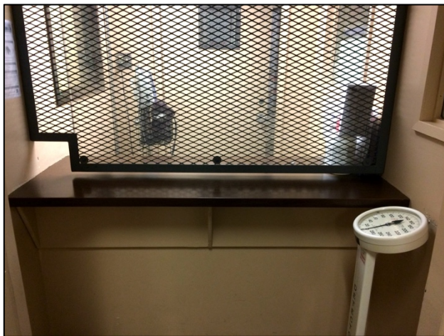
Figure 2: Examination room with insufficient space and compromised privacy
