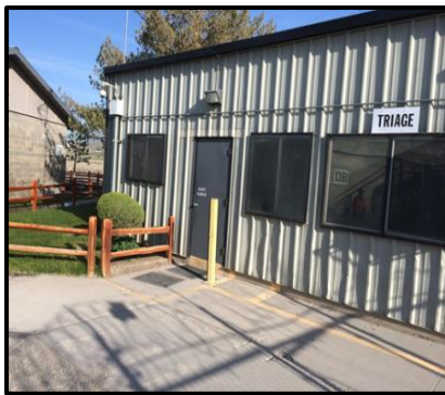
Figure 4: No protection from inclement weather
